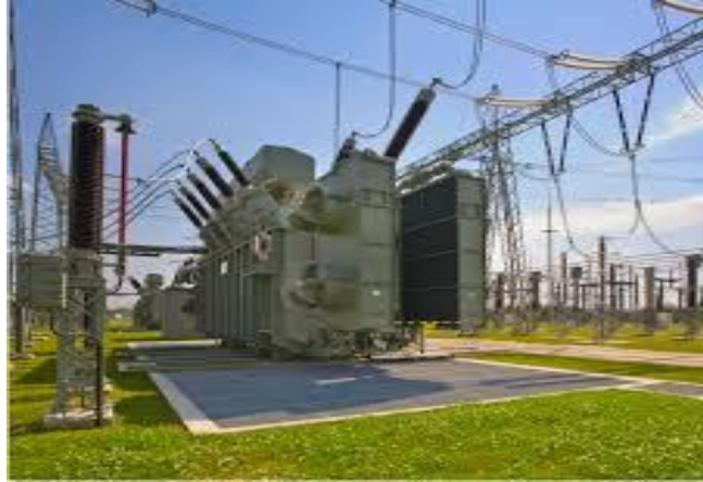
Figure2.8 Photo of a power transformer [4]
