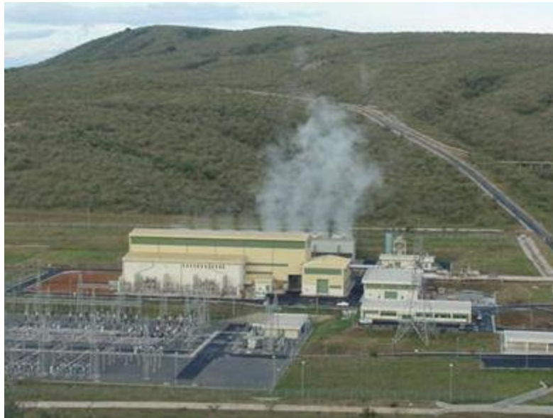
Fig 2.7 olkaria II power station
