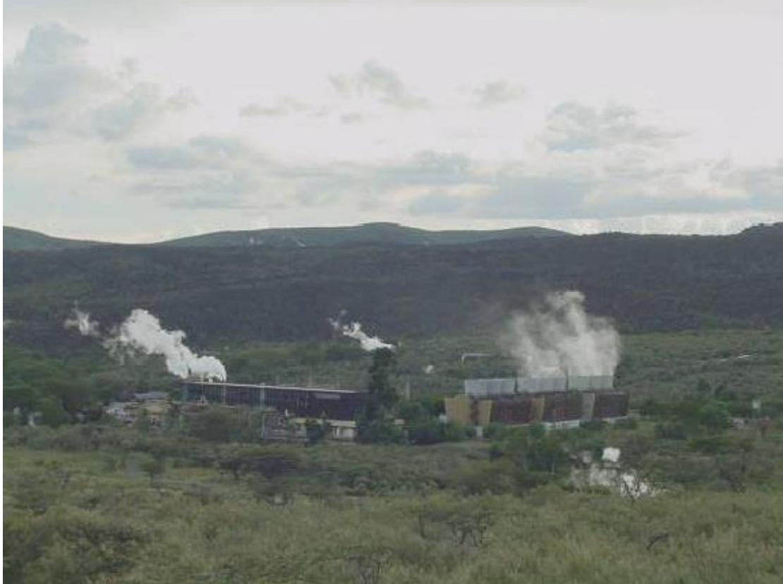
Fig 2.6 olkaria 1 power station
