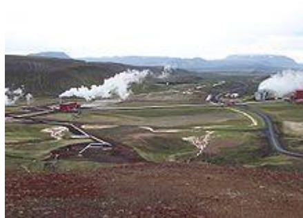
Fig 1.4 Krafla Geothermal Station in northeast Iceland (Source-google images)
