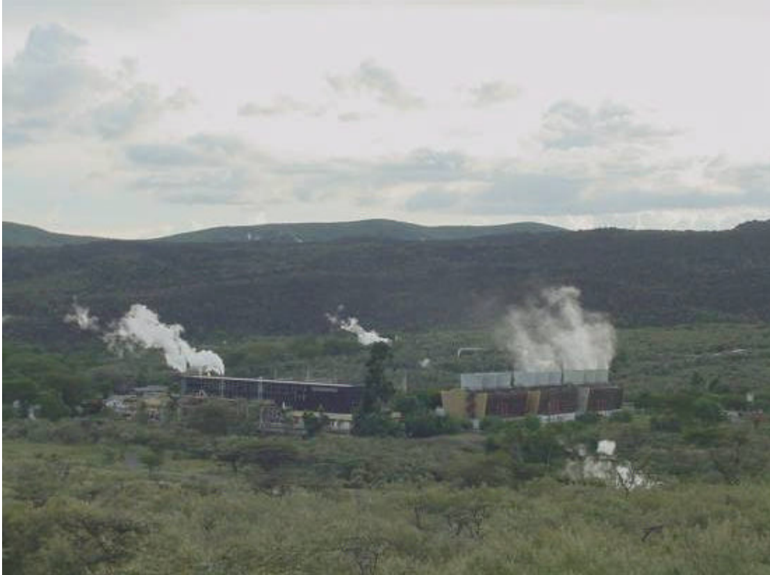
Figure 4.1: View of Olkaria I Power Plant
