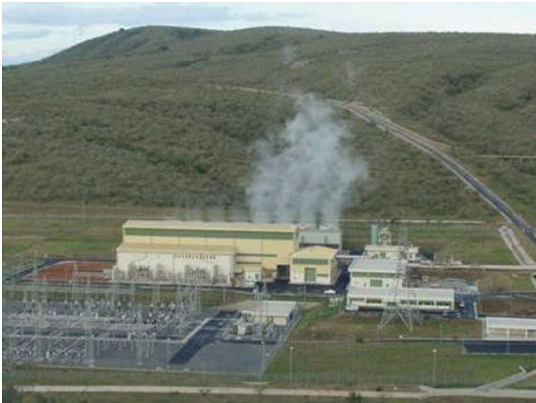
Figure 4.2: View of Olkaria II Power Plant
